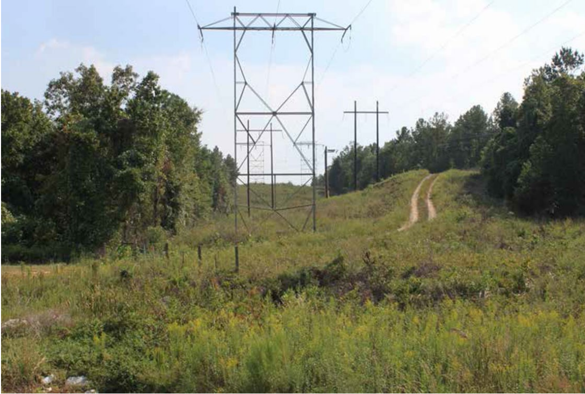
Figure 8. Ground view of utility swath/corridor (#3) in Figure 5
