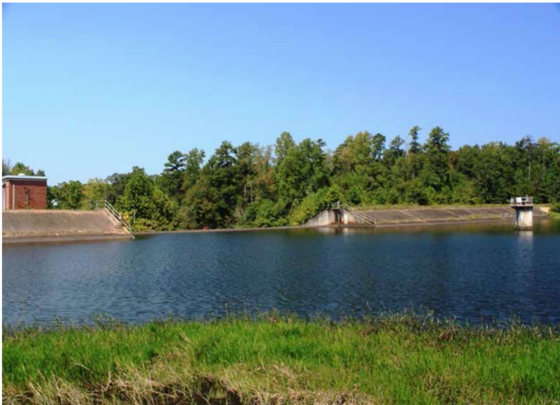
Figure 7. Ground view of the dam (#2) in Figure 5
