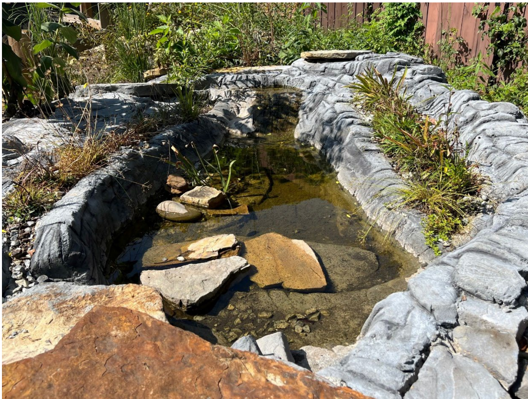
Figure 24. Functioning spillways enable ponds to fill to the appropriate level
